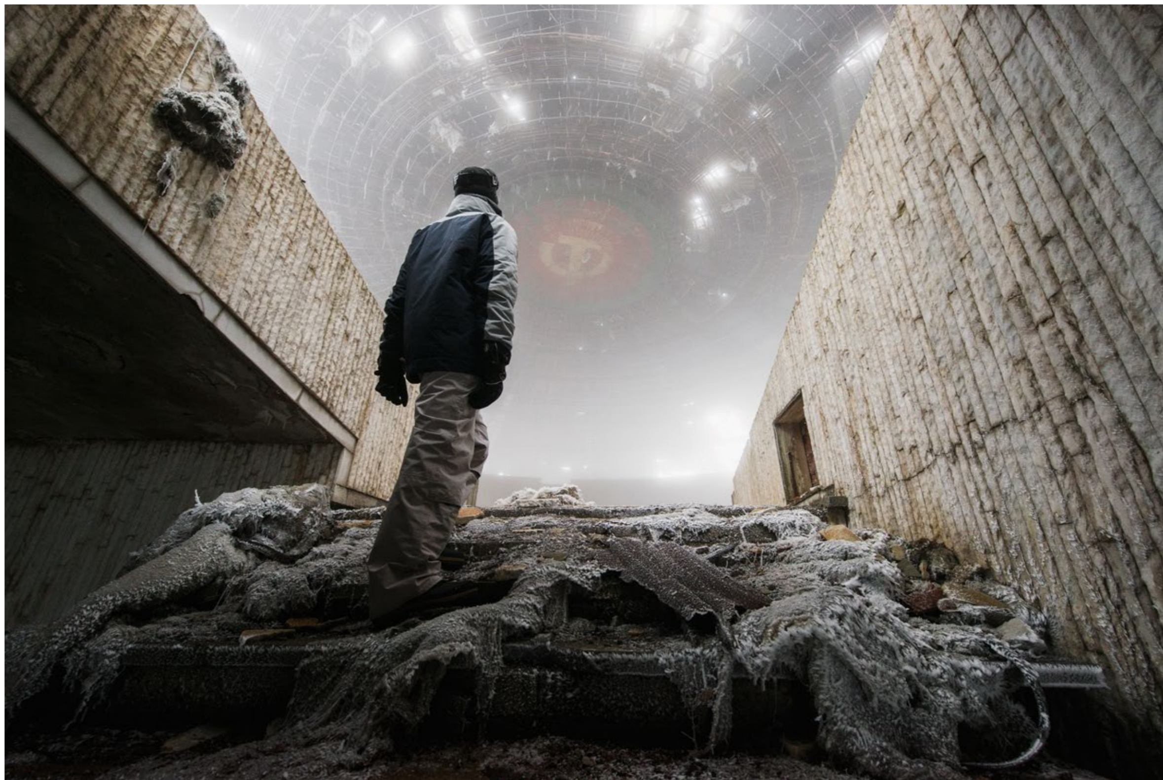
Self portrait taken inside a giant communist relic, Buzludzha, in Bulgaria. The saucer-shaped monument rises to a height of 107m. It now stands abandoned and vandalised. Nikon D800 with 14-24mm Nikkor lens. © Reginald Van de Velde
